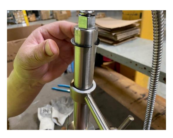
Once support arm is all the way down to white plastic ring, add black plastic clip slide it down to top of support arm. The black plastic clip, secures the support arm from moving.
