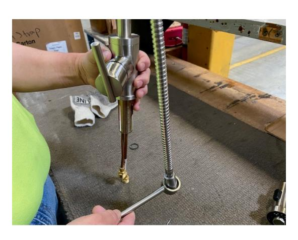
• Before installation make sure to remove sprayer and spring out.
